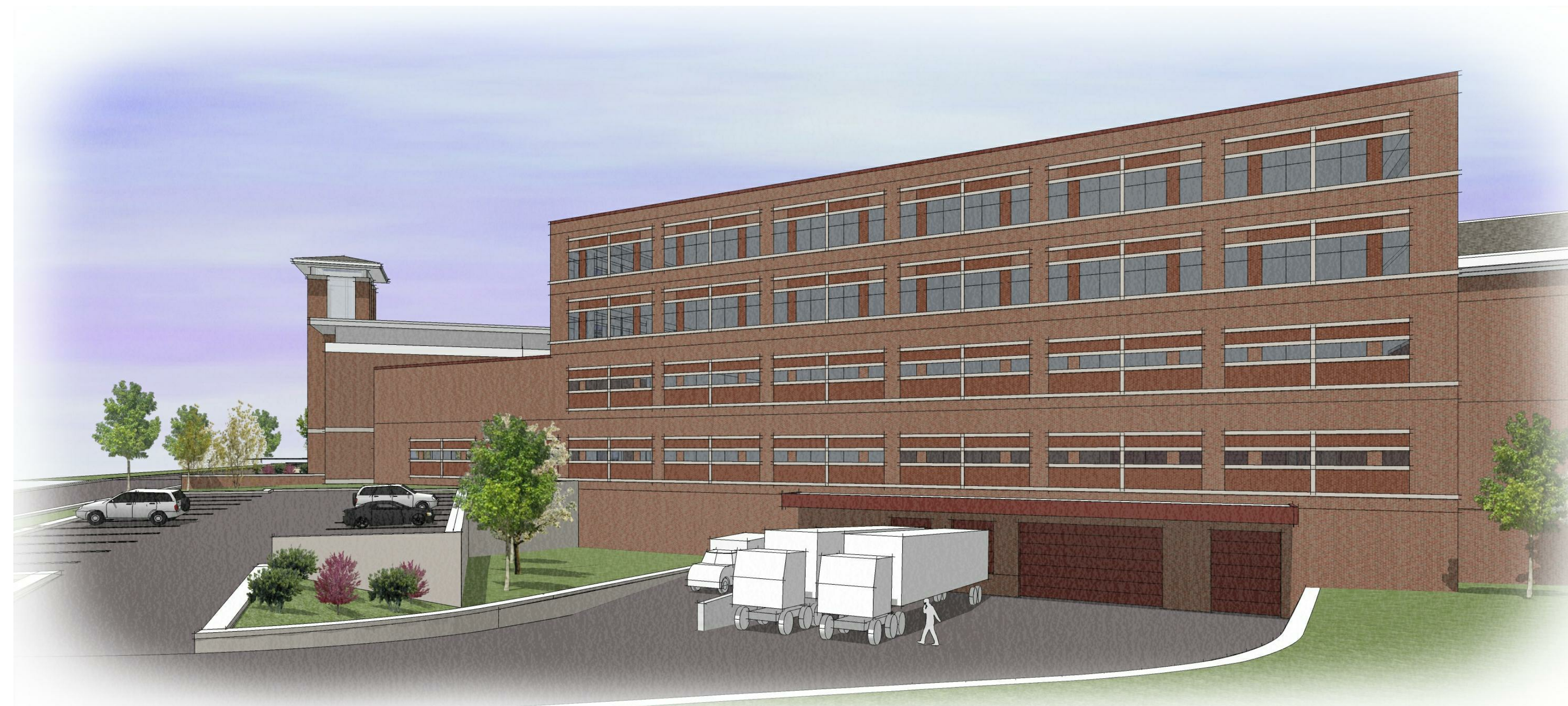
PEDESTRIAN VIEW OF LOADING DOCK
