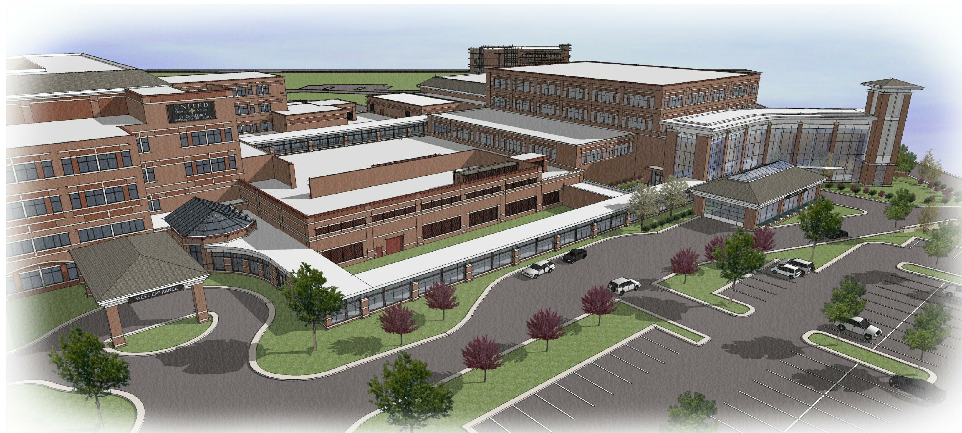
BIRDSEYE VIEW LOOKING SOUTHWEST
